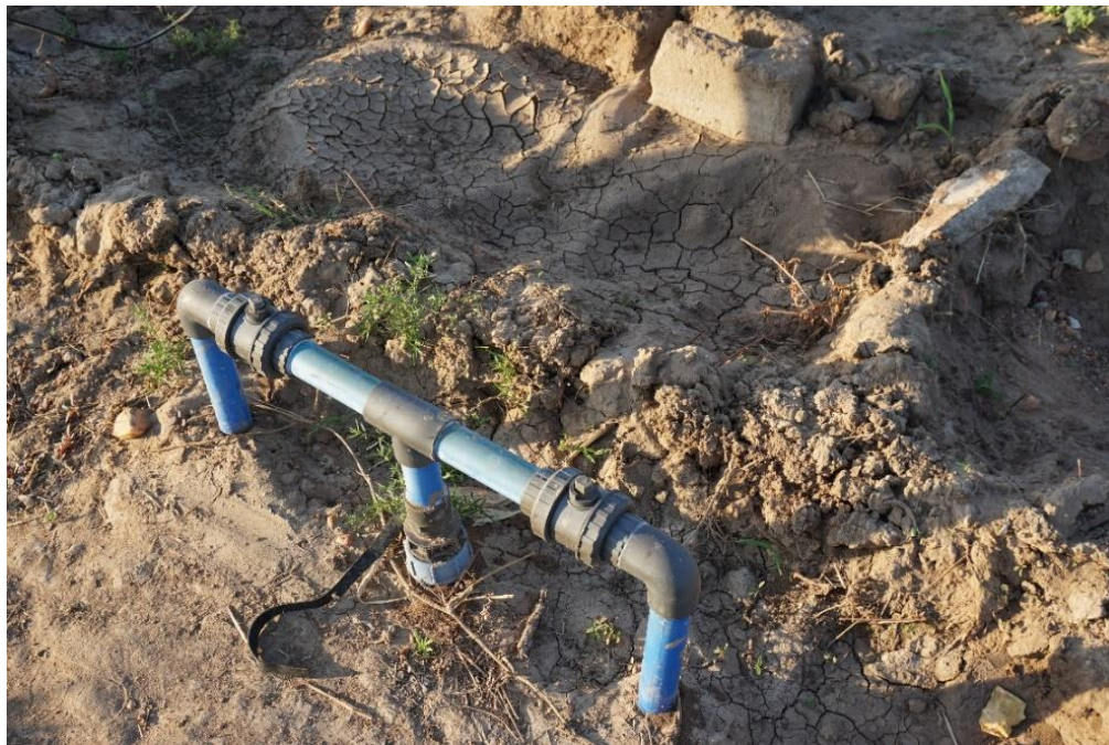
Figure 11: Valves – At points throughout the whole agricultural plot valves like this allow for the control of water flow in the greater system.
