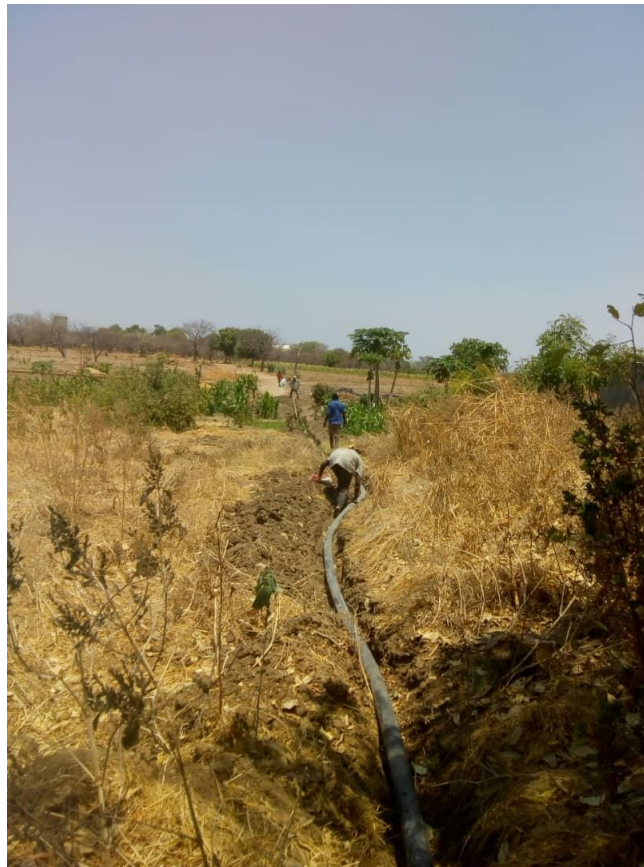
Figure 17: System Improvements – As we incorporated old and new piping into the system, time was taken to assess and repair the tubing that runs along the agricultural plot. Any damage here results in sections of the dripline system becoming inoperable.
