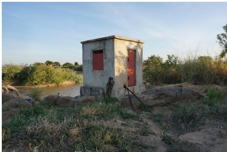
Figure 6: Pumphouse – This building houses the electric pump, protecting it from the elements and other dangers.
