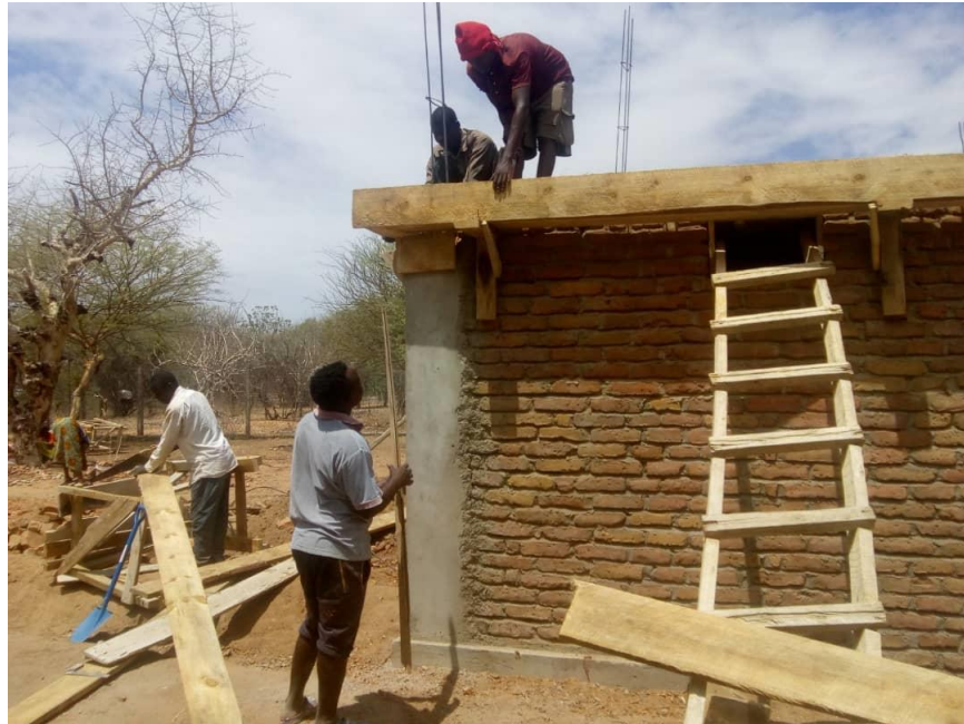
Figure 19: Reservoir Structure (b) – cement is incorporated into design to strengthen critical points.
