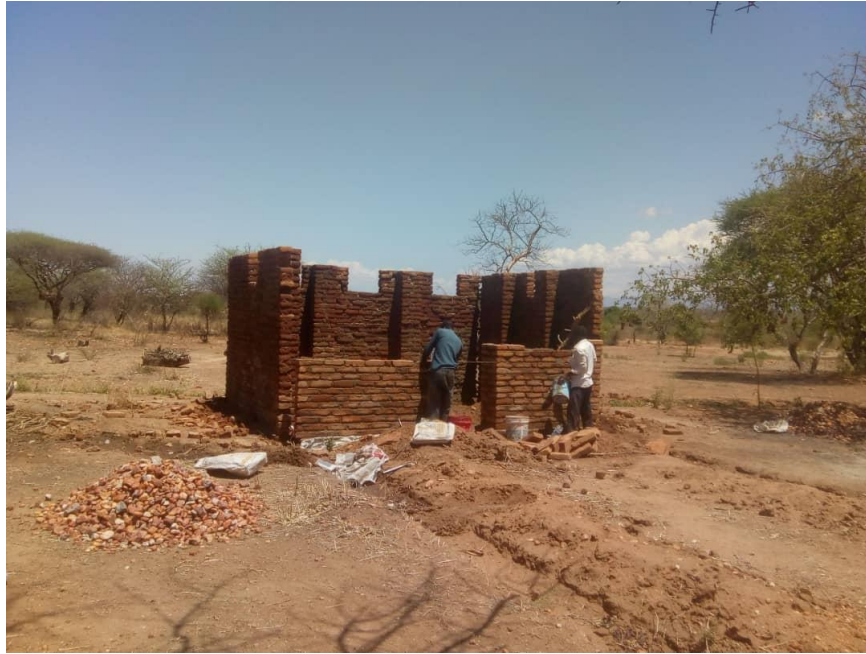
Figure 18: Reservoir Structure (a) – Local bricks made from crushed stones and clay form the walls of the structure. Pigs can be housed inside the structure as a source of manure. The roof will hold two 10,000 L tanks.
