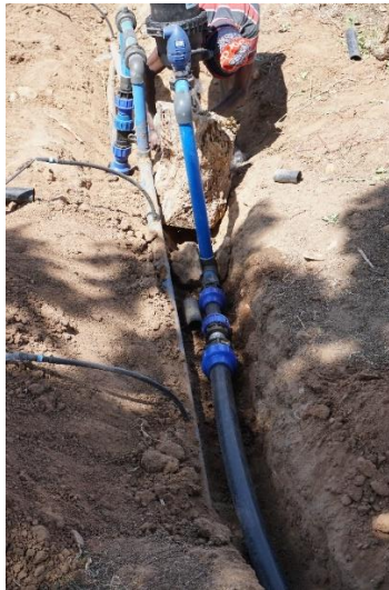
Figure 13: Varying Diameters – The tubes and pipes that connect all components of the system change diameter at certain connections, like the filter and driplines. The properties of the fluid changes with the pipe diameter.
