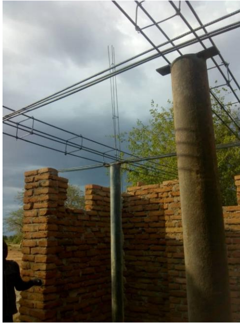
Figure 20: Reservoir Structure (c) – more cement pillars and metal rebar further strengthen the roof. The roof must support 20,000 L, 22 tons of water at max capacity.
