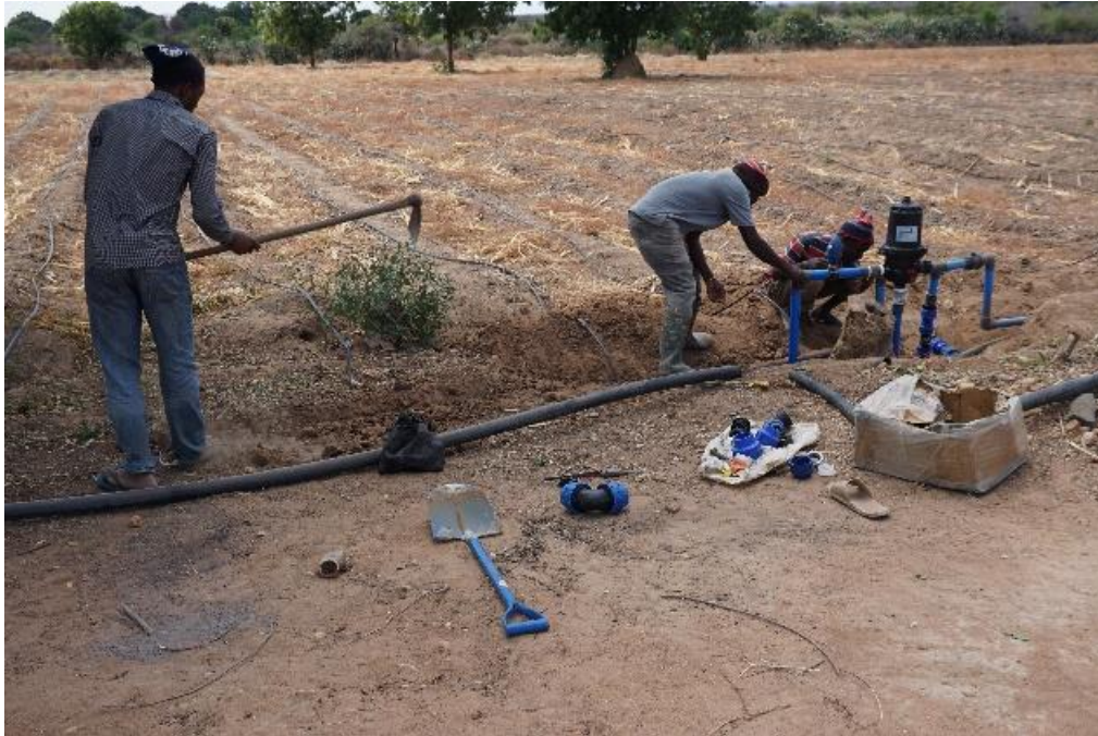
Figure 10: Filter – It is positioned at the intersection of which the water arrives at the plot. There is a drop in pressure that occurs as the water passes through it.
