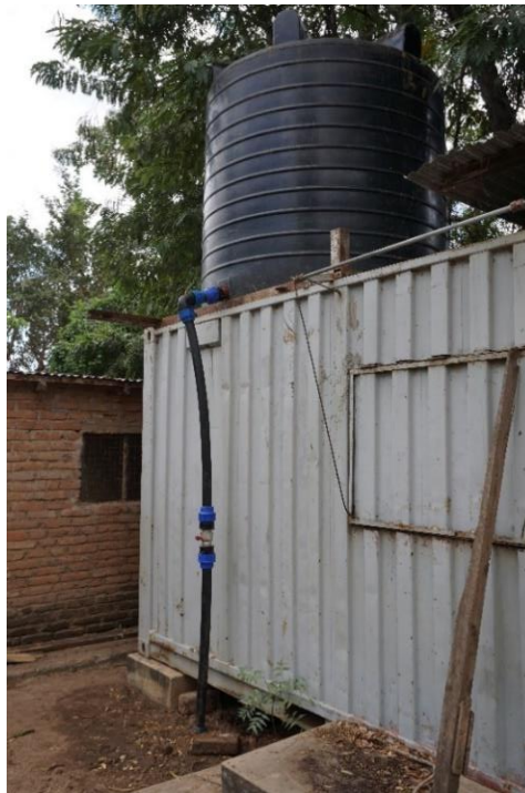
Figure 8: 5000 Liter Reservoir – Notice that an existing steel cargo container was used to provide elevation.
