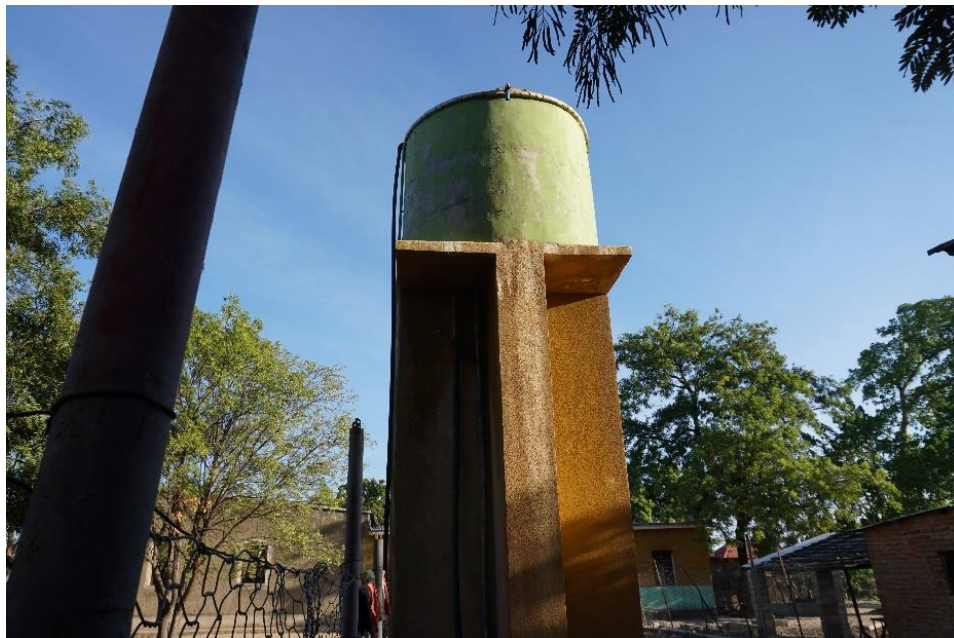
Figure 23: Concrete Water Tower – This tower stands ~9 meters high. It is the primary tank for the plumbing in the mission compound.
