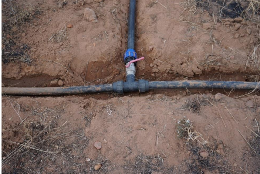
Figure 16: Main-line Source – the red valve opens and closes the connection to dripline field. At this T-intersection the pump is to the right and left, uphill, is the mission compound.
